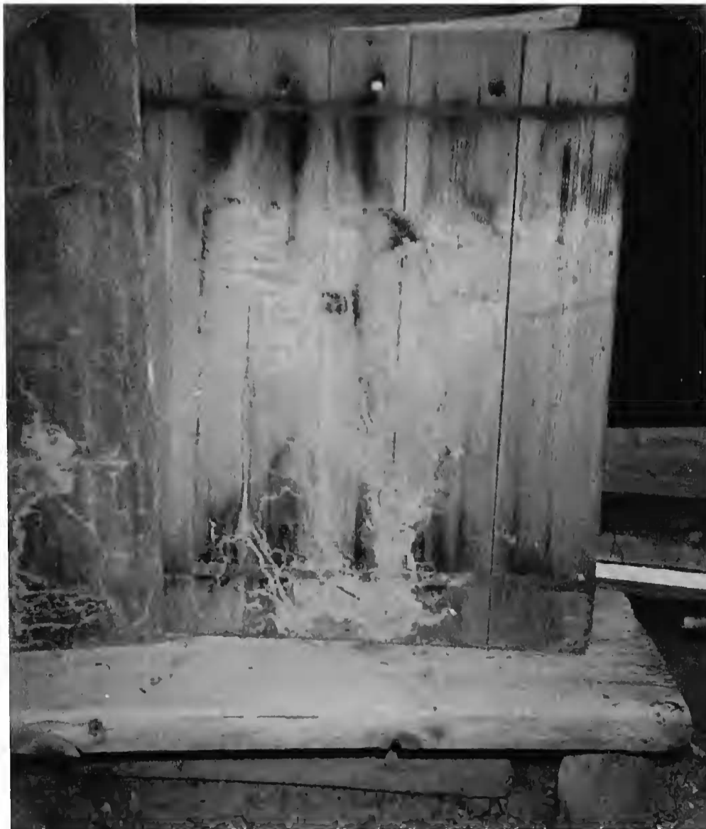
Figure 1. Surface scarification of wood caused by Gnathamitermes perplexus .
